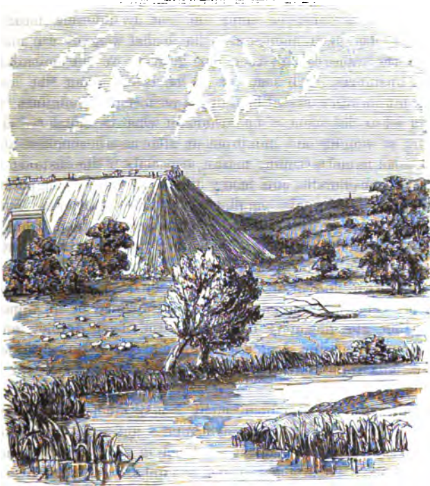
MAKING AN EMBANKMENT.
